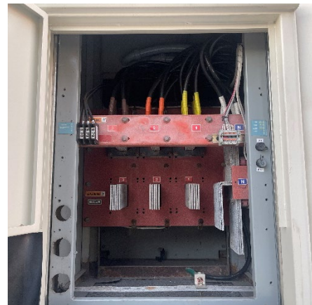
Buss Bar, Shore Power & Customer Connections
