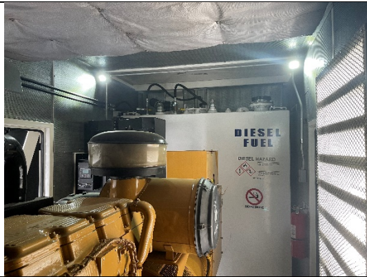
LED Interior Lighting
