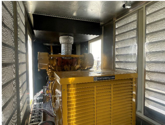
LED Interior Lighting/New Insulated Silencer
