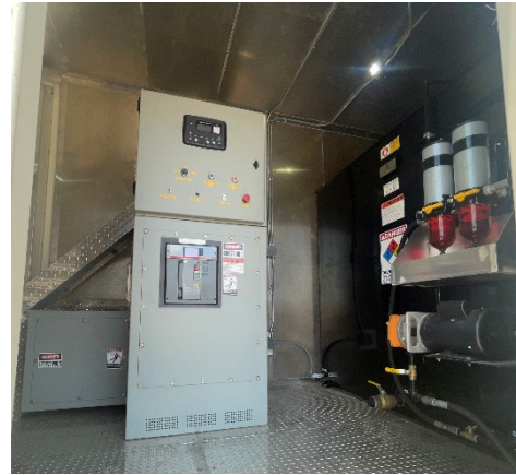
New UL Cabinet with Deep Sea 8610 Paralleling Capability 1200 Gallon Double Wall Fuel Tank
