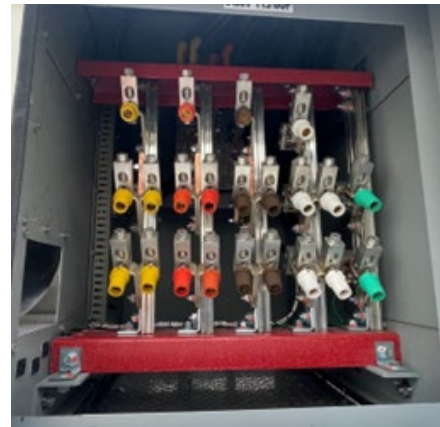
480V SmartBus with Cam Lok & Lug Connections
